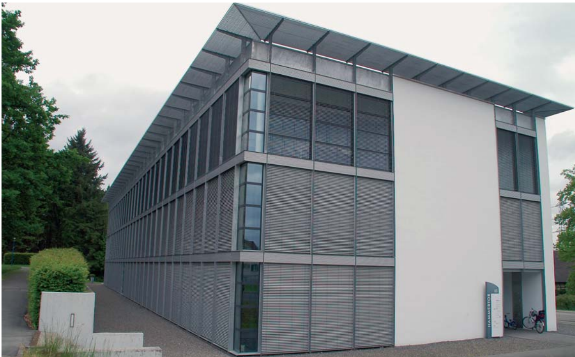
This is exemplary: the blinds are closed automatically at the weekend and at the end of the working day.
