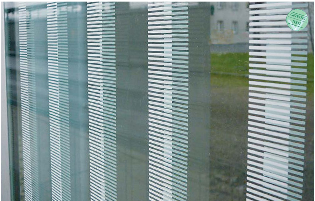
Details of the above wall. The pattern - columns of 2 cm wide stripes with 10 cm spacing between columns - is printed on both sides of the glass and in some places on the reverse is somewhat more liberally applied, which increases the 3-D effect on approach.
