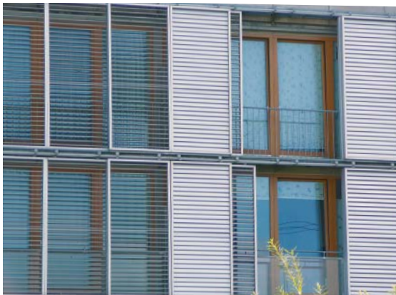
These horizontally movable blinds protect from overheating and avert bird collisions.
