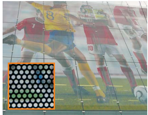
Printed sheets can be used to cover entire façades with effective advertising. Most are perforated with small holes and so permit an external view.
