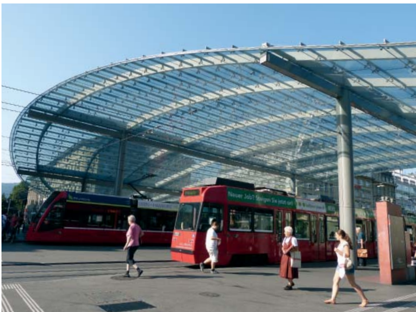
In general, such large glass ceilings are unproblematic. There is a slight risk posed by the edges, as they have a steeper gradient. Thanks to a point grid pattern over the whole surface, which also provides some glare protection, this danger has been removed.
