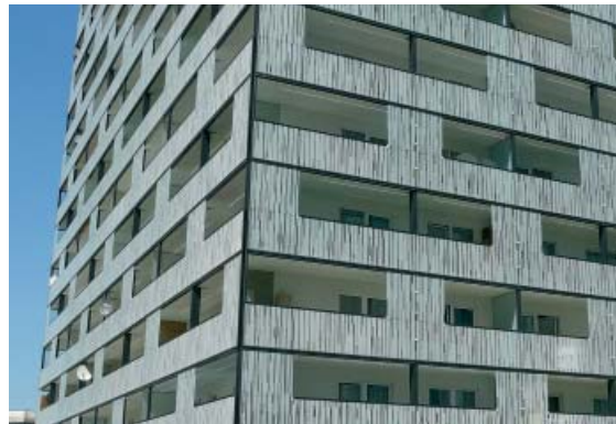
The screen printed pattern guarantees privacy for the terrace users and enhances the 3D structure of the building.
