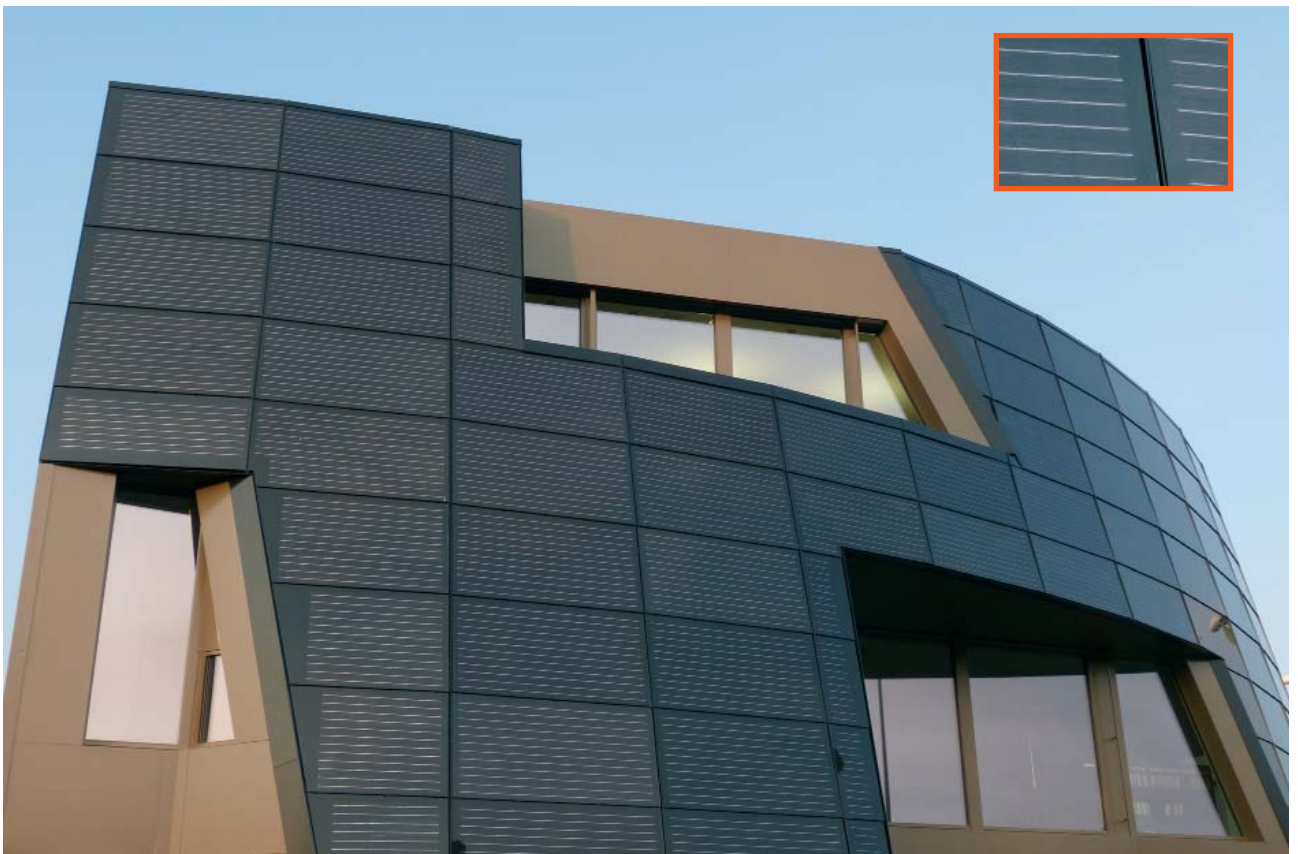
Innovative architecture with solar panels mounted on the façade. The solar panels are reflective, but the embedded lines delineate the structure and therefore they are not a bird hazard.
