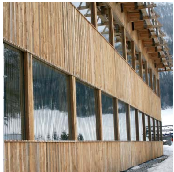
A good and cheap solution in this case: vertically tensioned nylon threads.
