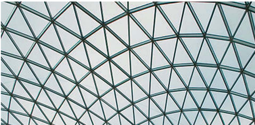
The triangular construction creates a lattice effect.
