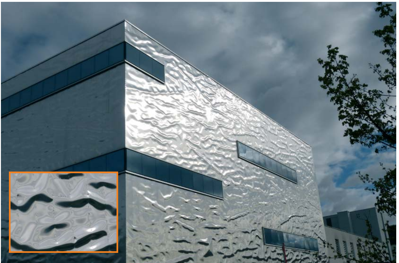
Although this warehouse is almost completely covered in reflective metal, the intense warping makes it harmless for birds.
