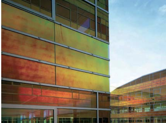
This strongly coloured, low reflective glass and the opaque corners make this building bird friendly.
