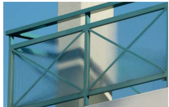
Semi-transparent balcony glazing, here made of moulded glass, is no danger for birds.
