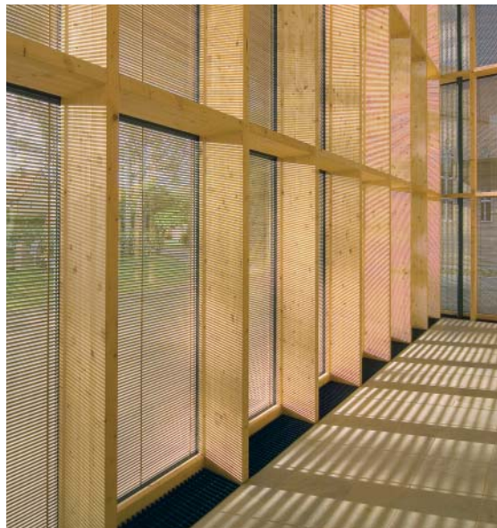
Double Glazing with embedded wooden blinds provides a lovely atmosphere.
