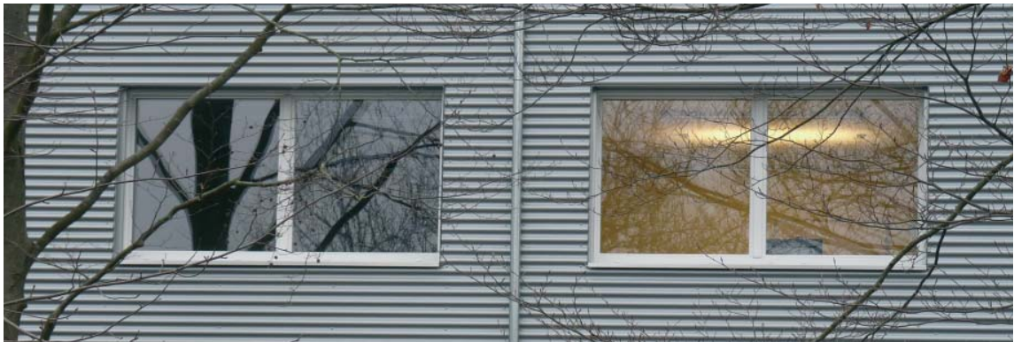
Reflectivity depends on a number of factors such as, for example, the lighting in the interior space behind. The same glass produces stronger reflections with increasing darkness of the background.
