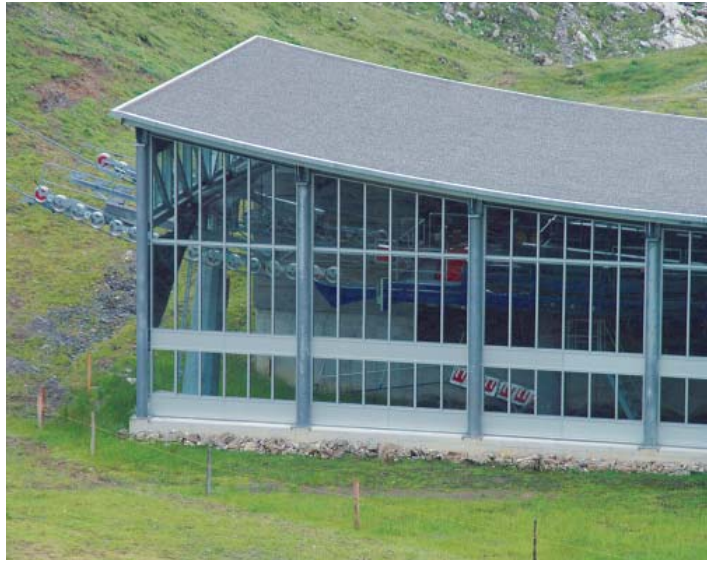
Valley station of a mountain cable car, glazed on three sides: birds fleeing late snowfall fly into the building and hit the windows - usually from the inside.
