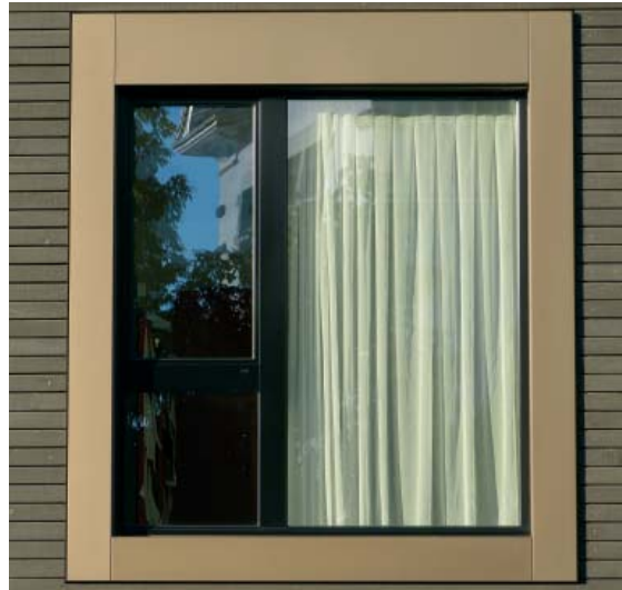
Light coloured curtains mounted close to the window reduce reflectivity: the difference is striking.
