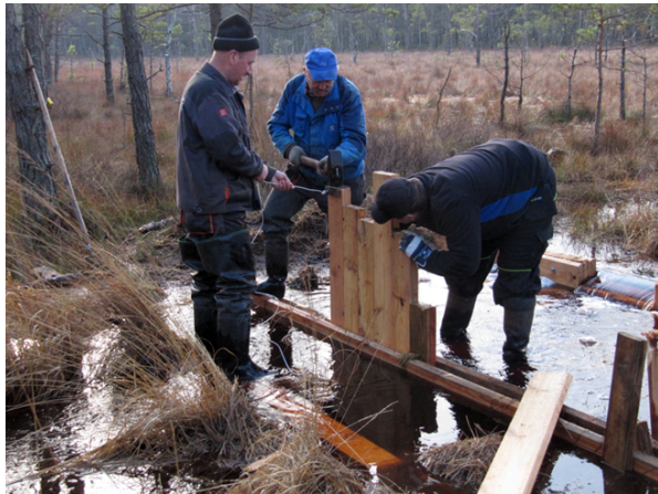
Ditches blocking in the Baltic bogs conservation project
