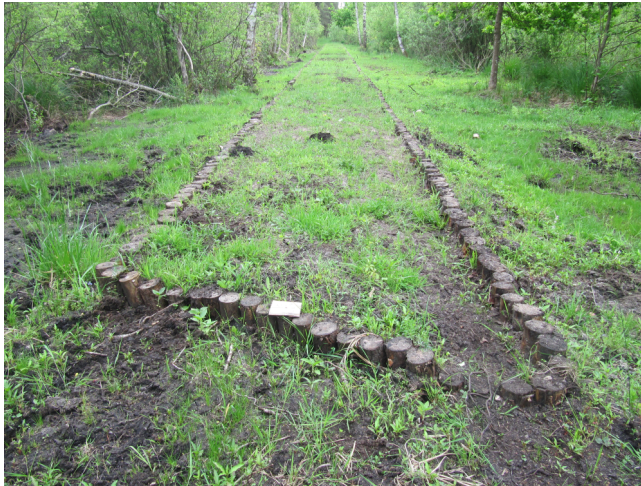
Peat dam strengthened by wooden elements. .
