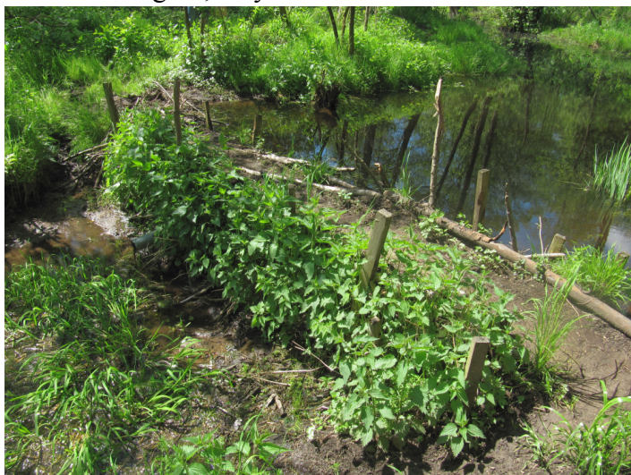
Mimic of beaver dam, developed by local farmer in Wielkopolska region, for maintaining water in the farm area
