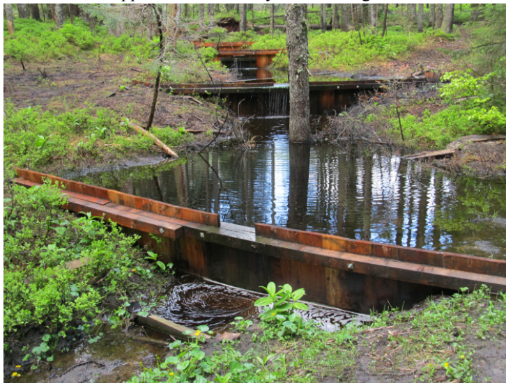
The “cascade” approach of ditches blocking is used also in other countries. Bog restoration in Austrian Alps.
