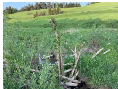
Beaver Dam Analog blocking drainage ditch in Bieszczady, using willow shoots - from building in autumn to the next summer. Photo credit: Andrzej Czech.
