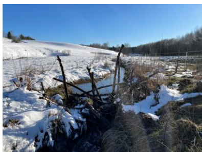
Beaver Dam Analog blocking drainage ditch in Bieszczady, using willow shoots - from building in autumn to the next summer. Photo credit: Andrzej Czech.
