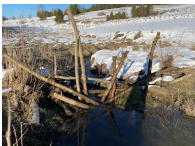
Beaver Dam Analog blocking drainage ditch in Bieszczady, using willow shoots - from building in autumn to the next summer. Photo credit: Andrzej Czech.
