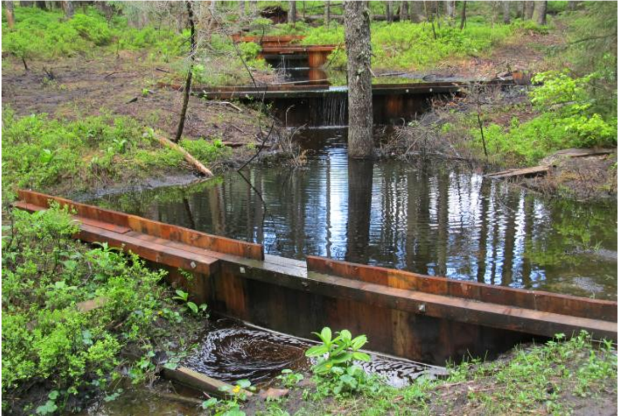
The “cascade” approach of ditches blocking is used also in other countries. Bog restoration in Austrian Alps.
