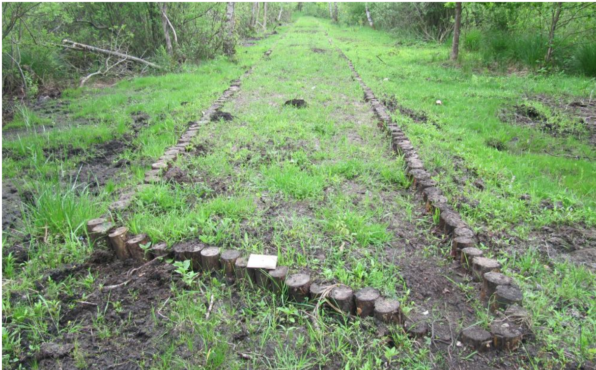
Peat dam strengthened by wooden elements.
