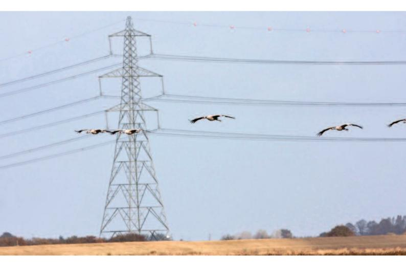
circuit. Short circuits can occur between phases (ie, from one wire to another), or to an earth source. Electrocution can also occur either by troops of small birds causing an arc or through the urination jets of large birds roosting on the cross-arms.
